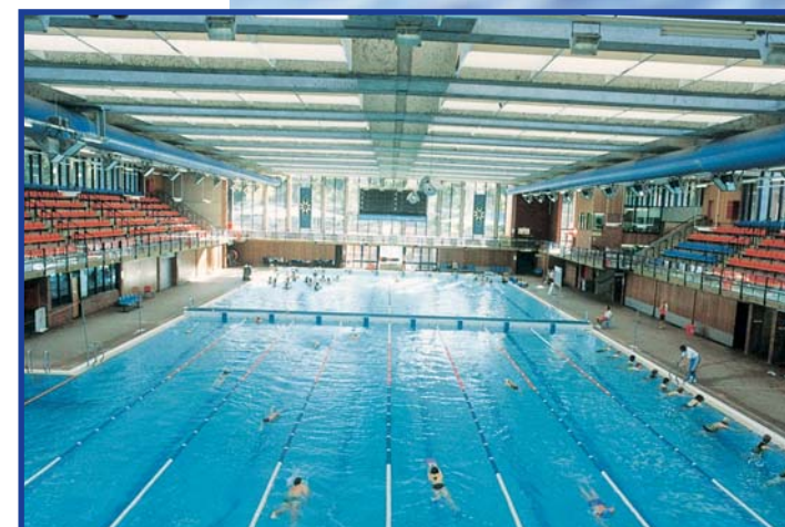
WARRINGAH AQUATIC CENTRE - Air to Water Heating
