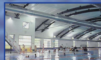
AUSTRALIAN INSTITUTE OF SPORT - Ground sourced heating
