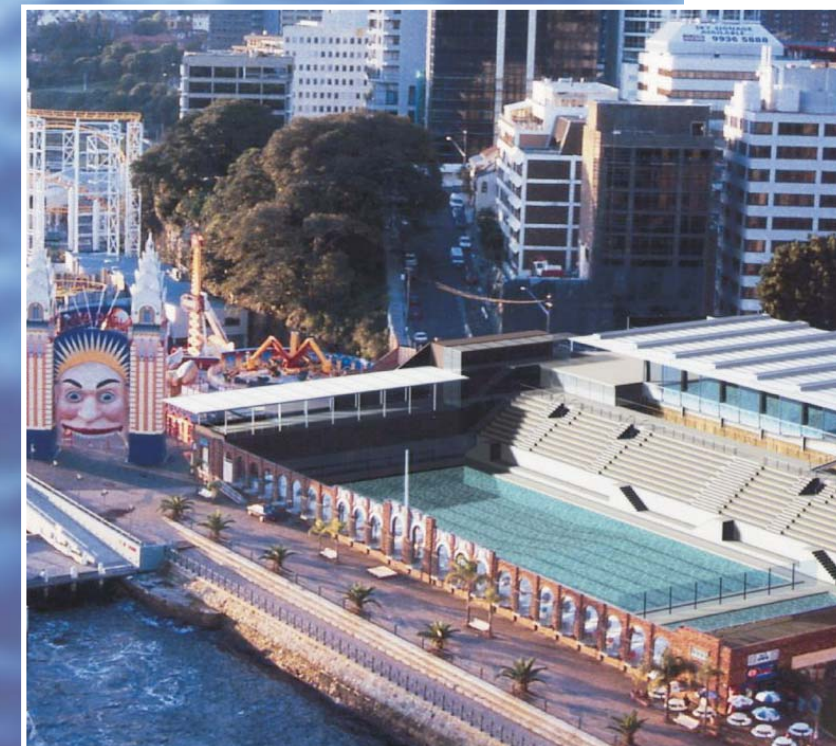
NORTH SYDNEY POOL - Water to water heating
